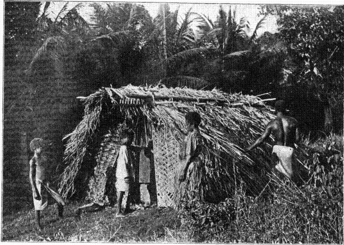
FIG. 56. ORIGINAL TYPE OF ANEITEUM HUT.
