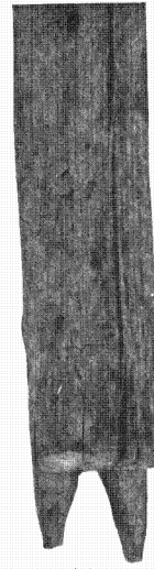
FIG. 79. UNDER SIDE OF LOWER END OF RAFTER.
