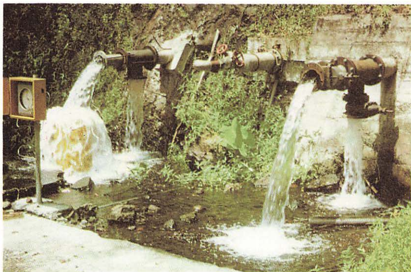
FIGURE 9.—Horizontal wells yielding water from a dike complex in Fautaua Valley, Tahiti. Photo by Michael Becker.
