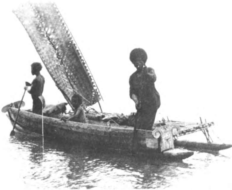
FIGURE 159.—Small waga with temporary coconut-leaf sail, Wagifa, Goodenough Island (photograph by D. Jenness).
