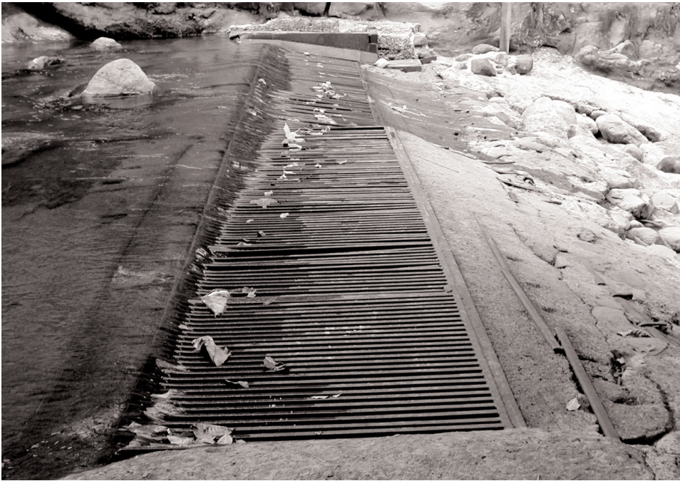
Figure 10. 'Āao Stream Diversion (below USGS Stream Gauge No. 16604500). Most stream flow is diverted into irrigation ditches.
