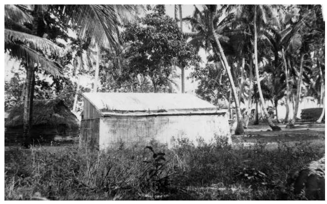
**Roll 62:4** Typical source of water supply on these limestone, springless islands, Lomati. Cement tank, with galvanized iron roof and gutters to catch the water. Ascended the plateau wall by the trail up from Lomati.
