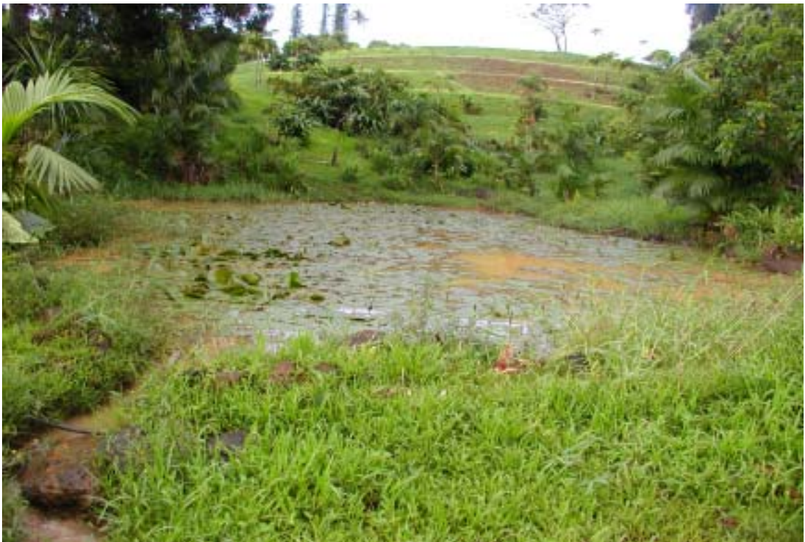
Photo 2. The banks of Pond 1 appear to be stable. Note turbidity from recent surface flow, water lilies and small streamlet connecting Pond 1 with Pond 2.
