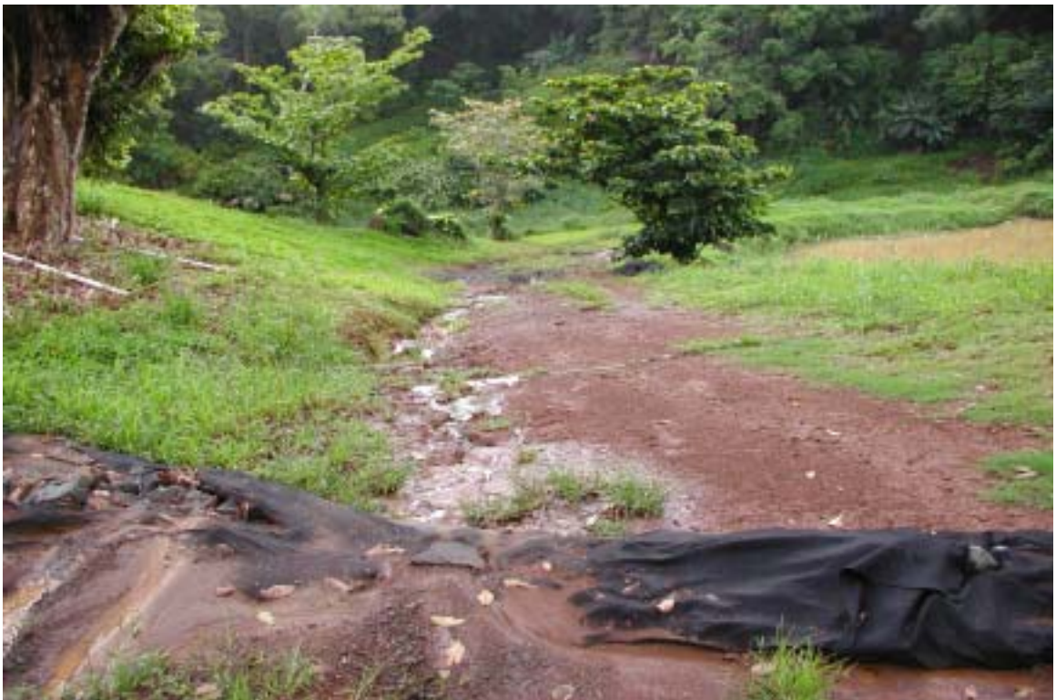
Photo 9. Erosion on jeep trails in Gulch 3. Note that the rock filter berm is ineffective in preventing erosion and sediment is carried over the berm toward Pond 6 and 7 (Pond 6 is in the background on the right side).
