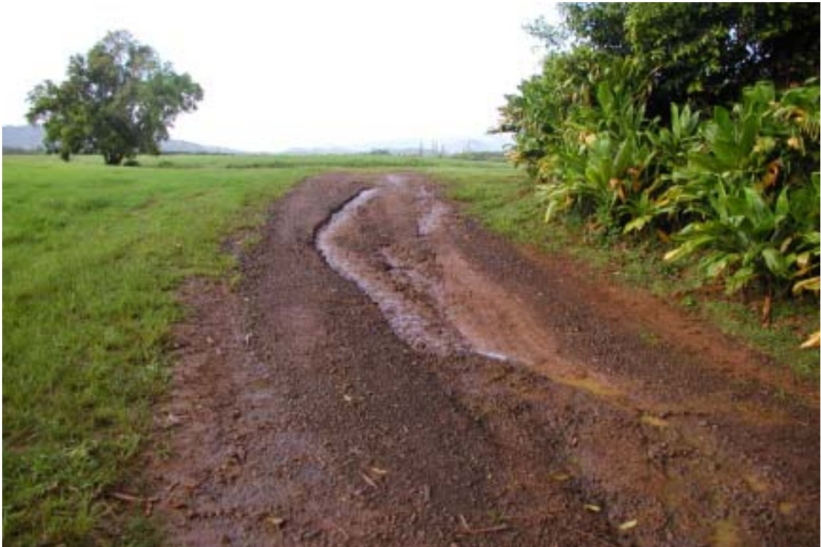
Photo 11. Erosion on jeep trail in Gulch 3 up gradient of Pond 1. The gravel is ineffective in protecting the trail from erosion, and the 18" CMP culvert under this jeep trail near Pond 1 is ineffective at handling storm flow.
