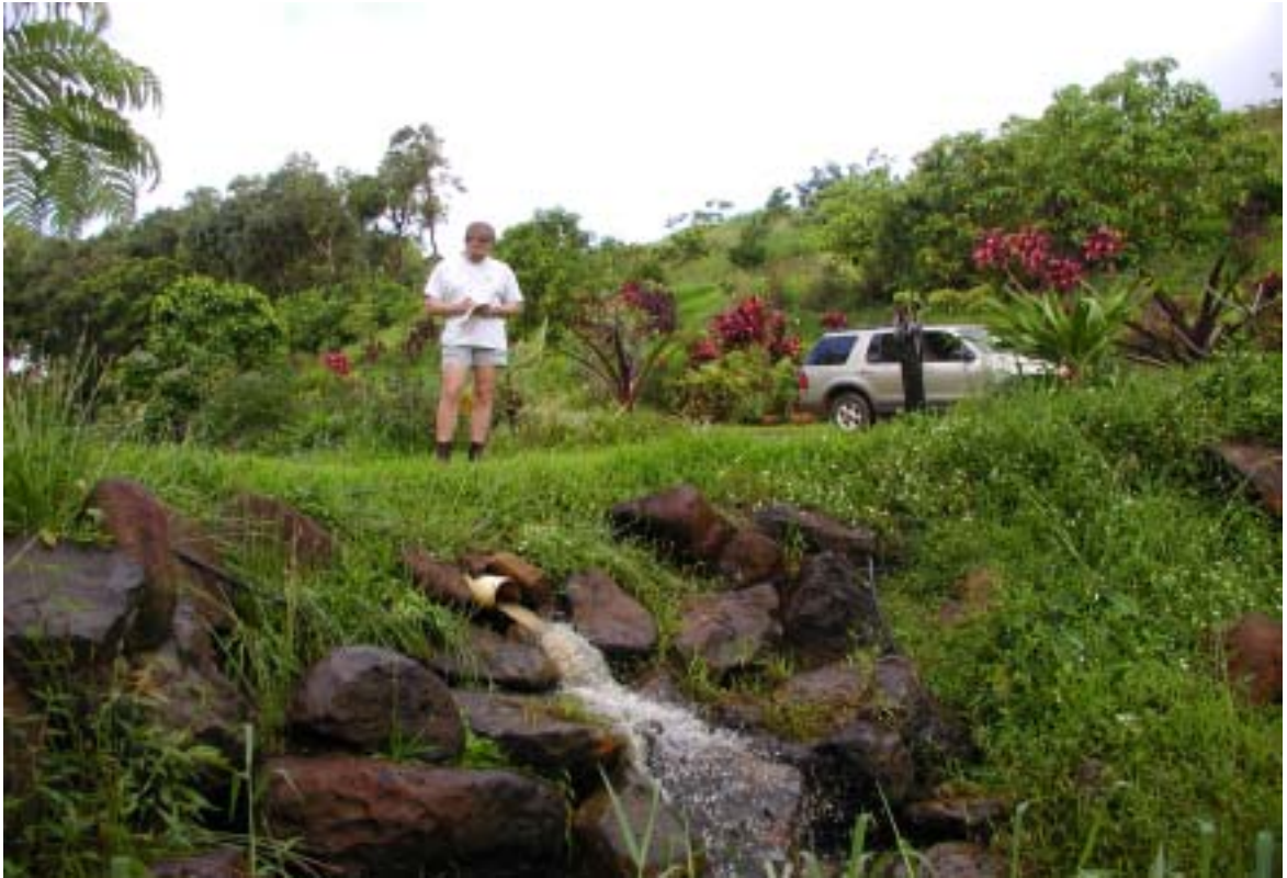
Photo 3. Six-inch PVC discharge pipe form Pond 2 into Pond 3.
