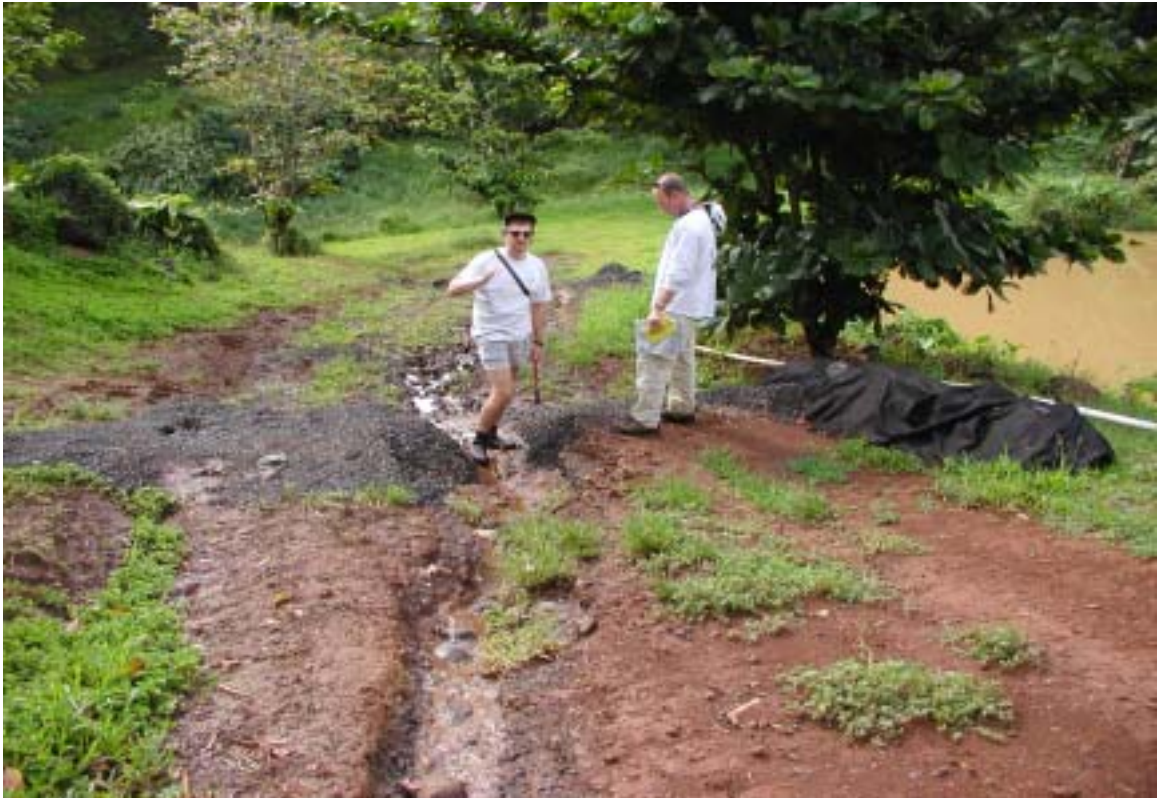
Photo 10. Erosion on jeep trails Gulch 3. Note that the gravel berm is ineffective and has been breached by concentrated runoff along the jeep trail. (Pond 6 is in the background right side).
