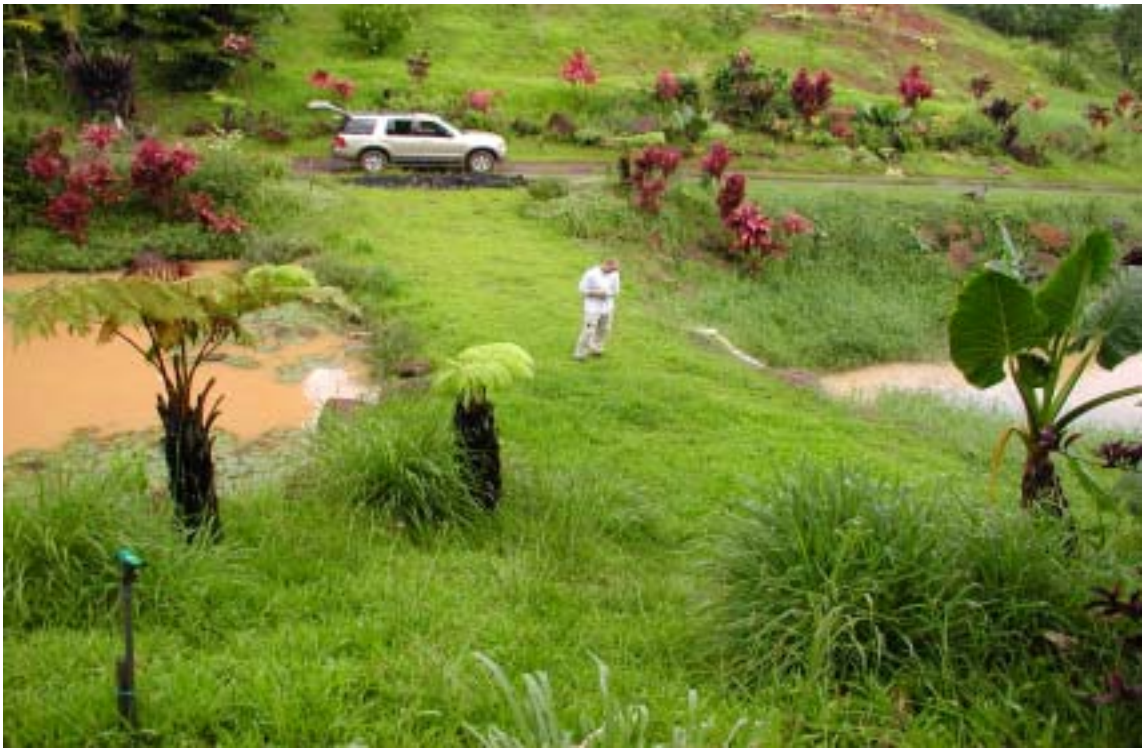
Photo 1. The landscaped areas around Pond 2 and Pond 3 appear to be stable. Note the 6" PVC pipe connecting the ponds under the grassed causeway (Photo 3 shows a different angle of the discharge end).
