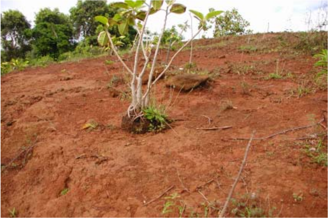
Photo 12. View of erosion on the bare slope close to Ponds 3 and 4 in Gulch 3. Over a half foot of topsoil has been eroded away as indicated by the exposed roots of the shrub in the center of the photo.
