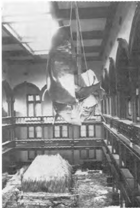
An old house frame from Kaua'i set up by Hawaiian house builders undergoes final thatching with pili grass. It is one of two traditional houses surviving in Hawai'i. The whale overhead now has its papier-mâché body. Photo attributed to W. T. Brigham, 1901.
