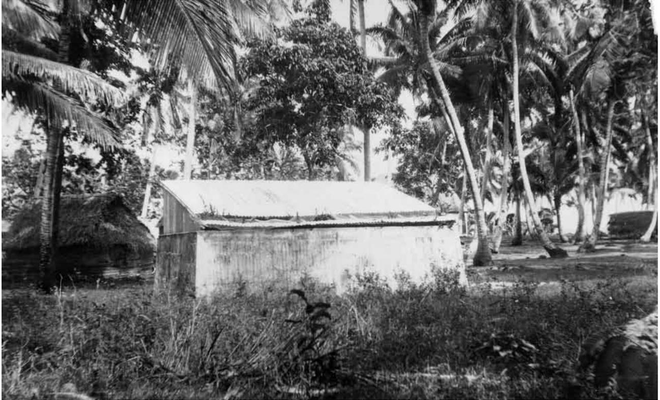
**Roll 62:4** Typical source of water supply on these limestone, springless islands, Lomati. Cement tank, with galvanized iron roof and gutters to catch the water. Ascended the plateau wall by the trail up from Lomati.
